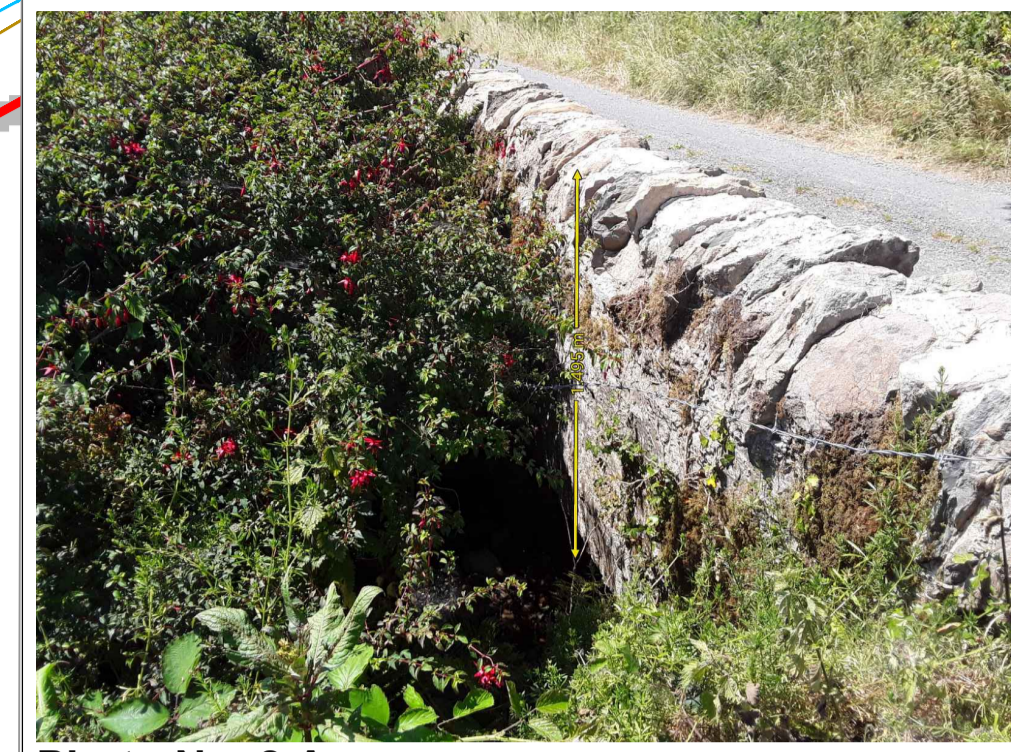
Photo No. 8 A
